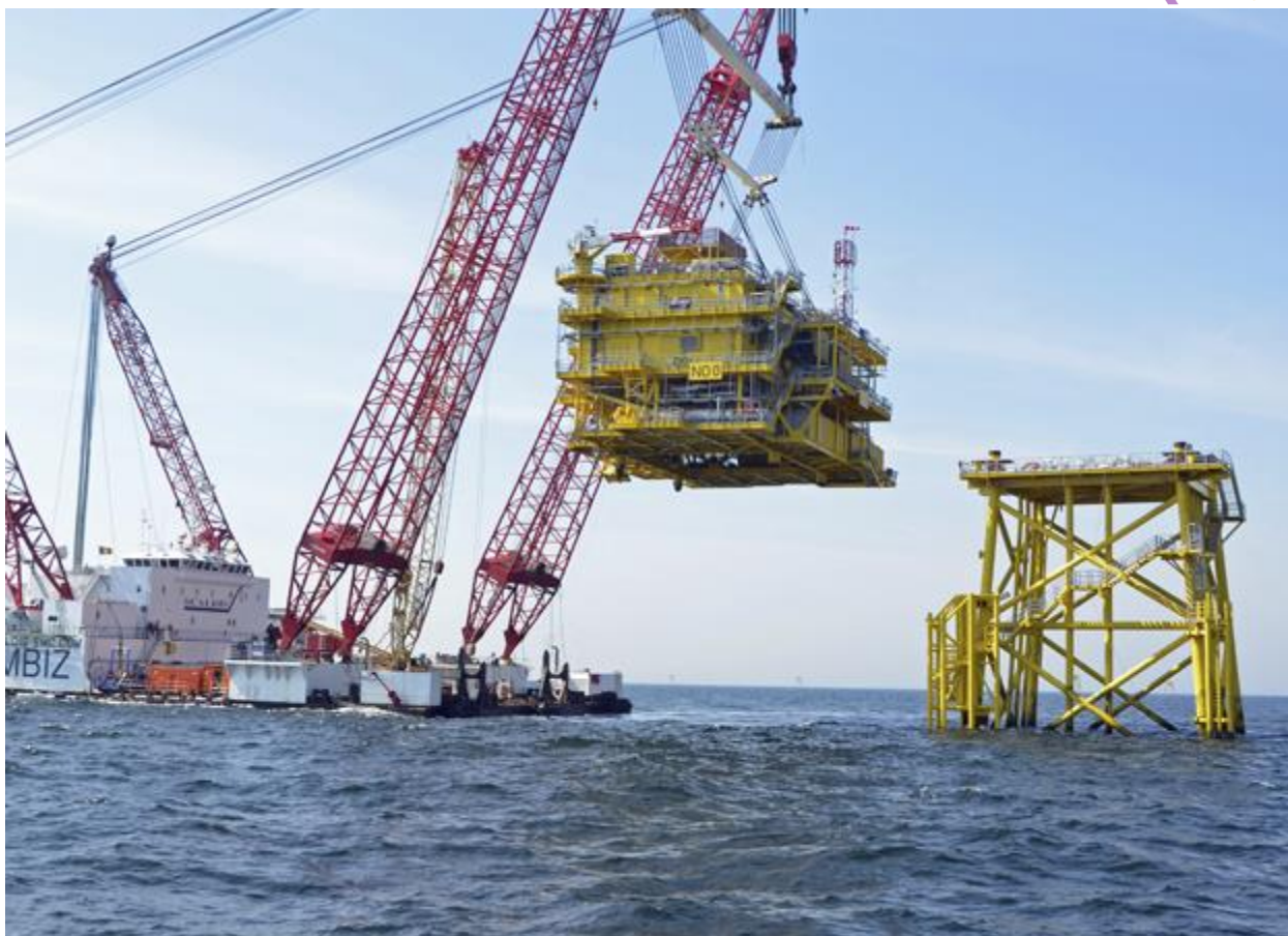
Figure 3: Installation of RWE's Nordsee Ost Platform
